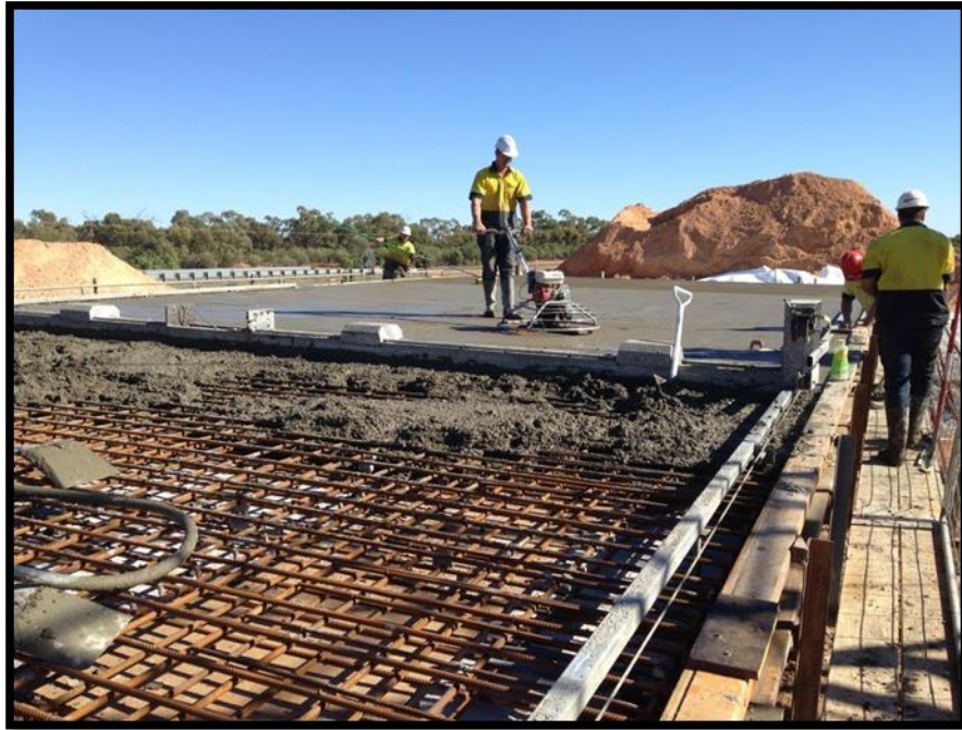
Cuttaburra NO 3 Bridge
