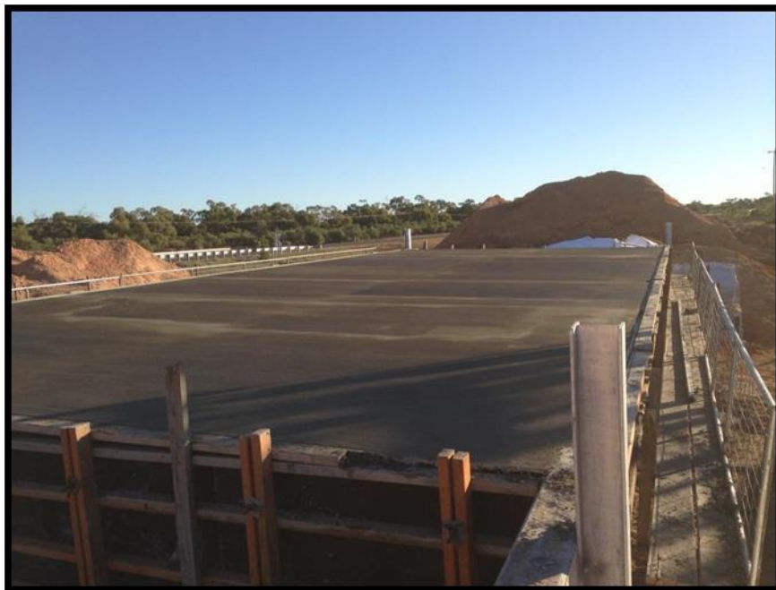
Cuttaburra No 3 Bridge
