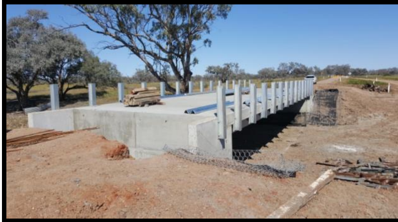
Whiskey Creek Bridge
