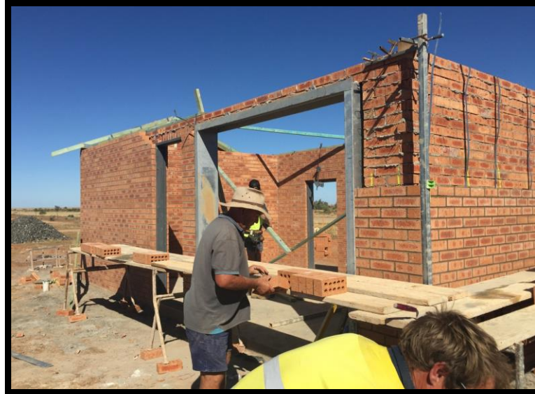
Walkden's Bore – construction of the pump house
