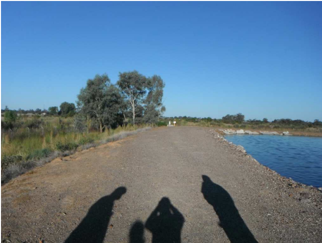
Figure 4.6a – Inlet pit EP3 (in distance) at STP
