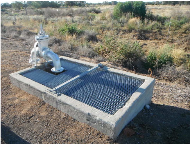
Figure 4.6b – Inlet pit EP3 (in detail) at STP
