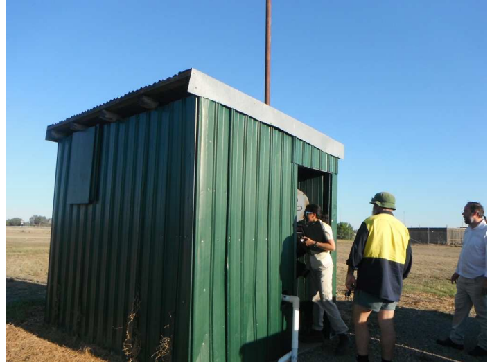
Photo 4.5b –Renshaw St SPS (SPS 7)
