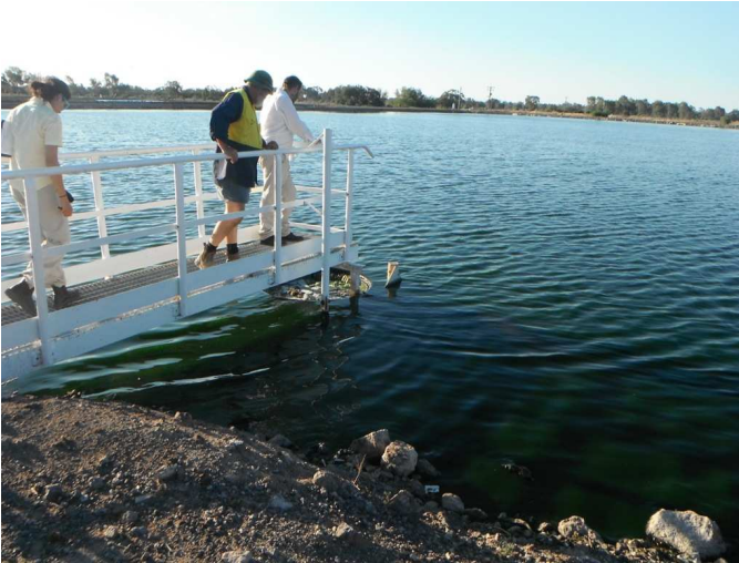
Figure 4.10 – Oxidation Pond No. 1 outlet
