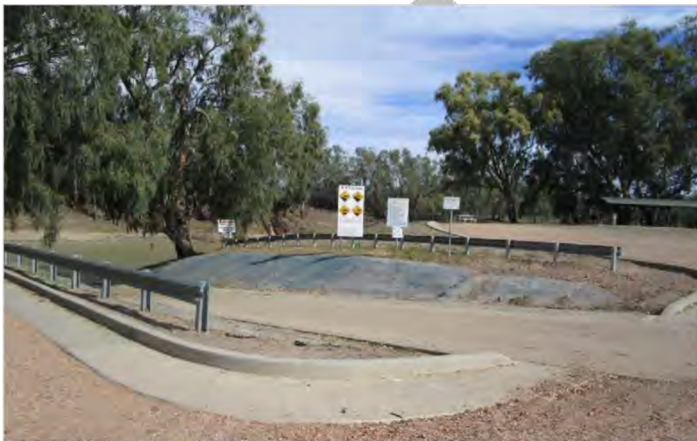
Reserve 78045: North Bourke Boat Ramp. Recent repairs & upgrades to ramp
