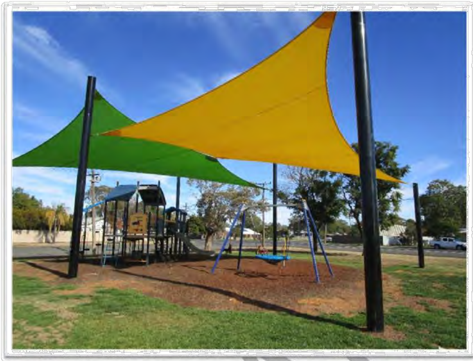
New playground works completed at Jones Park (2020)
