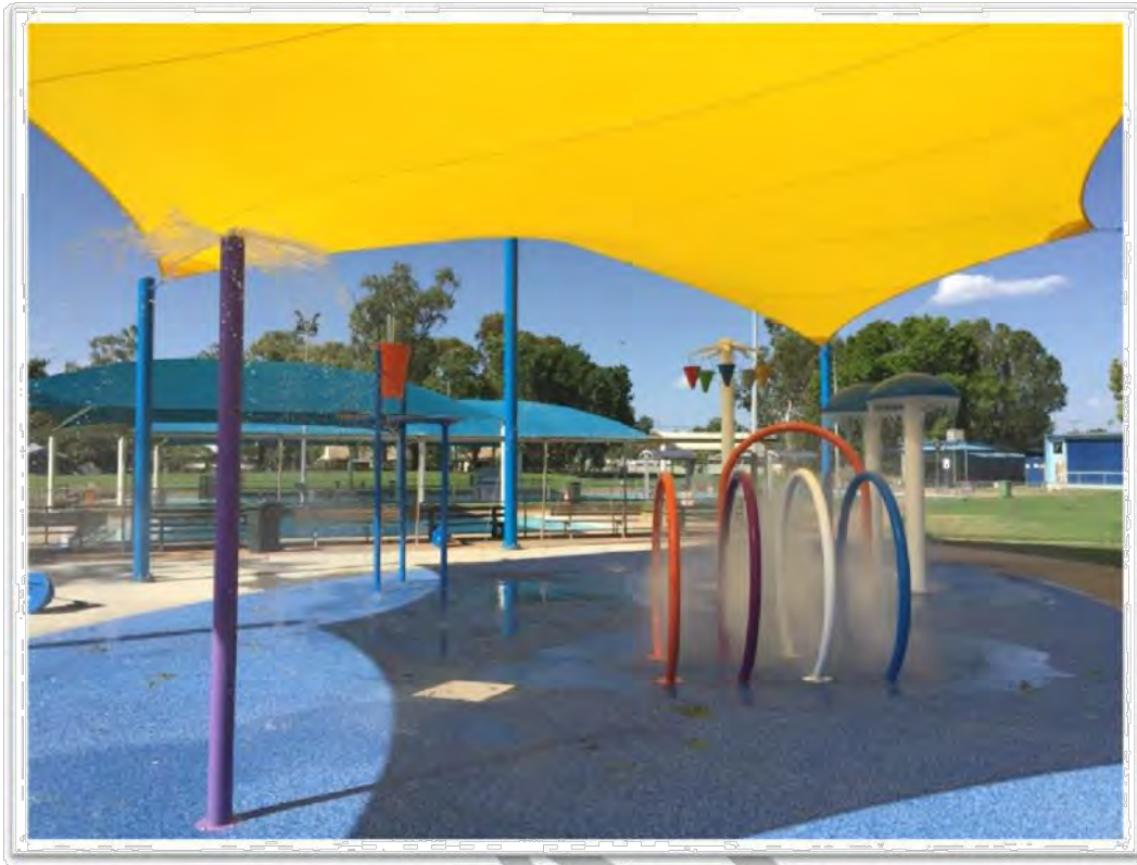
Bourke Pool improvements
