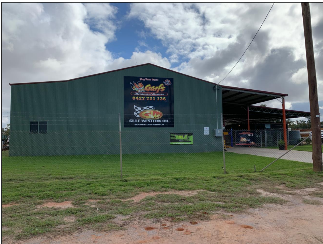
Figure 4. Image of Existing Business (photo taken 27 May 2022)
