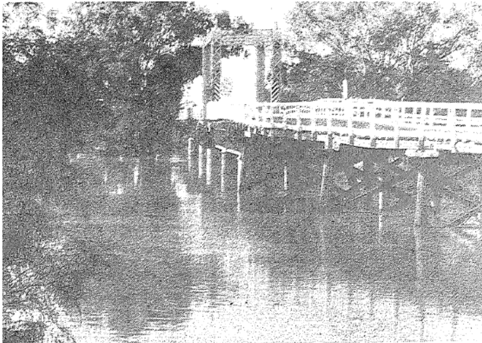
Plate 45 – Looking south-east across Darling River from immediately upstream of Old Bourke Bridge (image captured 17/05/1988). (Source: The Western Herald )
