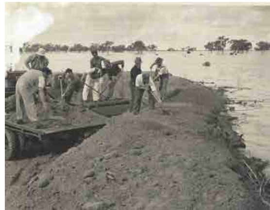
Plate 8 – Construction of levee bank. (Source: Council)
