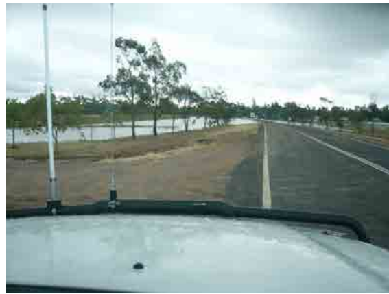
Plate 99 – Looking west from Mitchell Highway crossing of Bourke Town Levee. (Source: Council)
