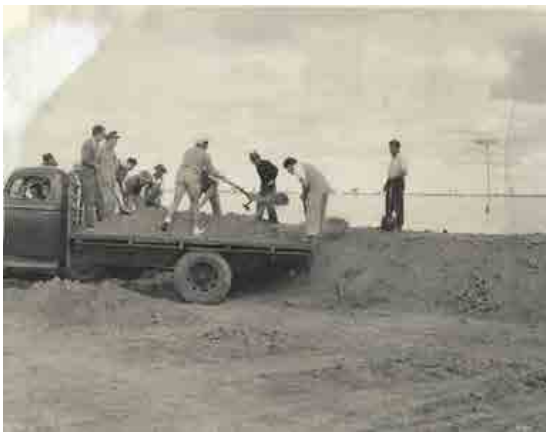
Plate 7 – Construction of levee bank. (Source: Council)
