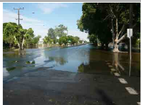
Plate 88 – Mitchell Street inundated to the west of its intersection with Tarcoon Street. (Source: Council)
