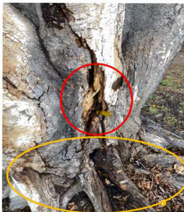
Figure 3 – Tree 3 with lower trunk wound, dead buttress roots(orange) and probe to 25cm depth showing extensive decay (red).
