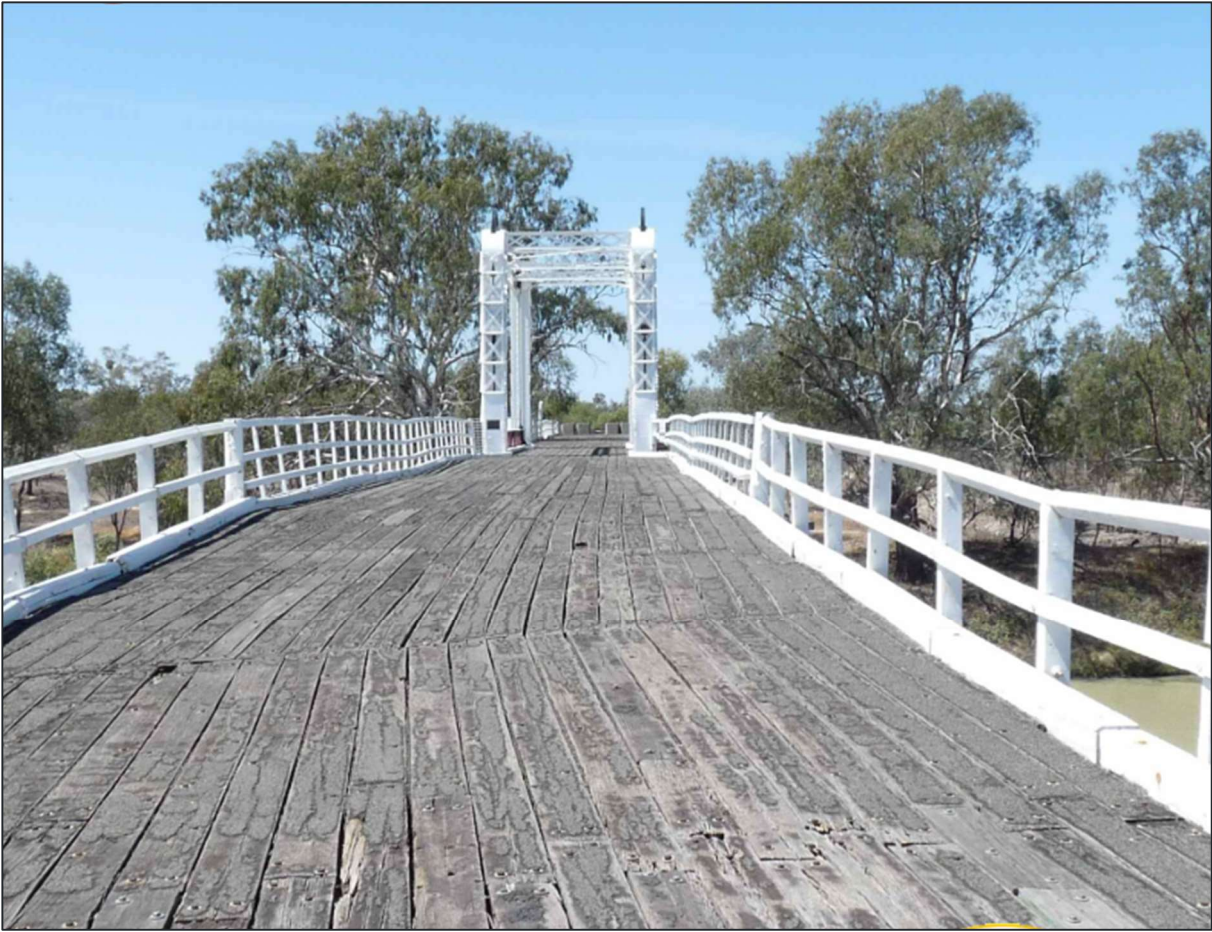
Figure 1-6: North Bourke Bridge Western Approach Source: FBE 2024
